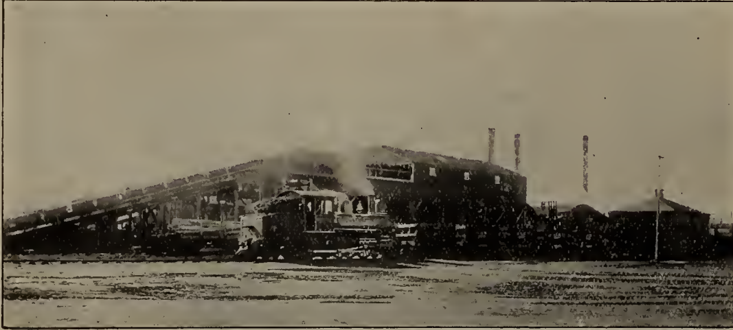
COLLIERIES AT WESTVILLE, NOVA SCOTIA.
